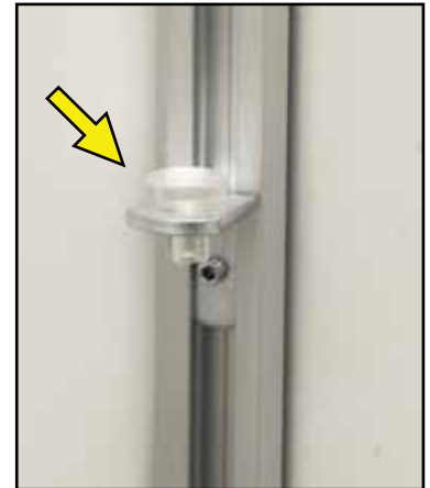
View showing Shelf Bracket installed along track.
