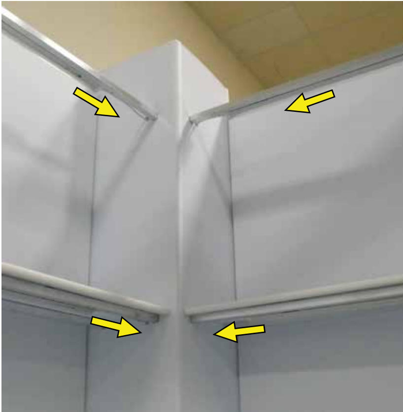
View showing typical Fluorescent Light installation along Booth.
