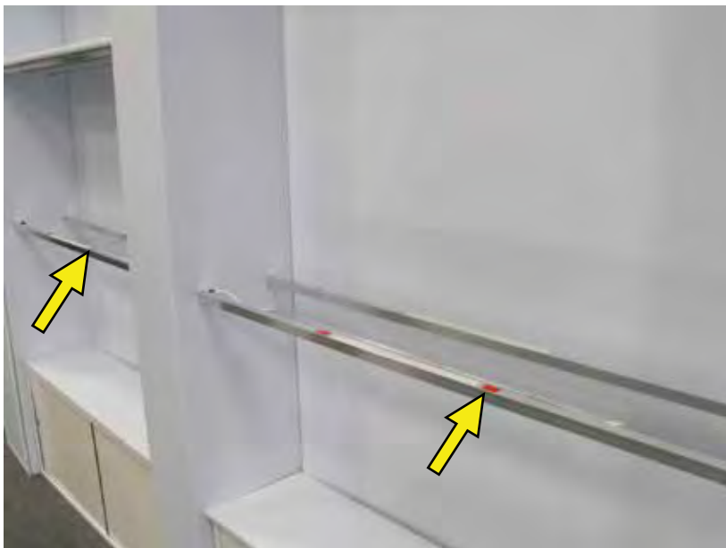
Red vinyl is placed along the front light support bars to assist in mounting the Fluorescent Lights.
