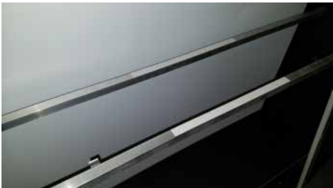
View of installed Support Bars
