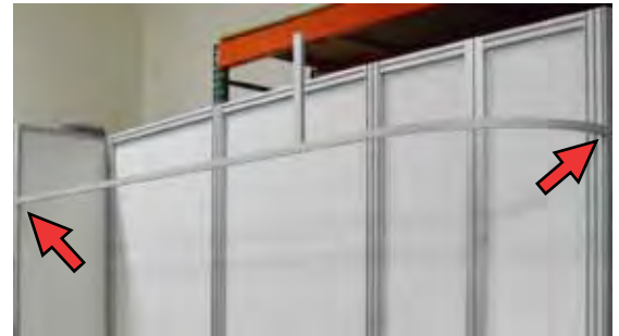
View showing Header Braces attached to Back Wall
